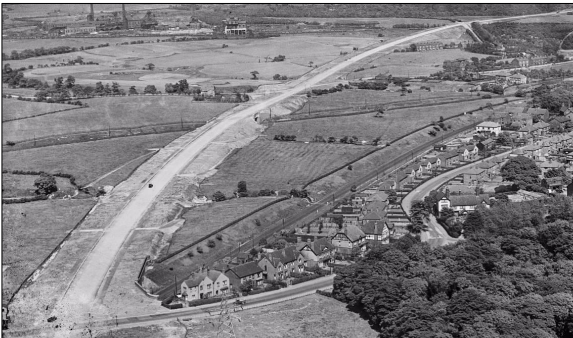
Plate 3: An aerial photograph of the site north of Lumber Lane taken during the construction of the East Lancashire Road across the existing railway lines in 1932.
